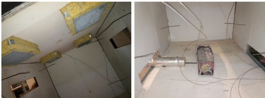
Figure 7. Position of samples under the ceiling, and the position of the burner
